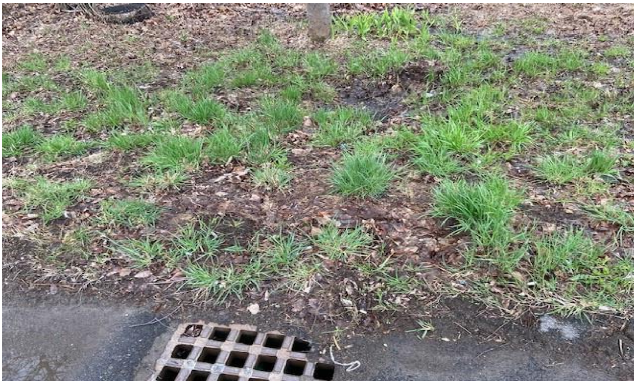
Photo #6 – Existing Catchbasins on south side of Pleasant Street
