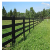
Fence for highway trail
